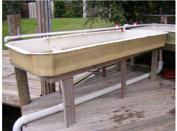
Water is piped in from bayou, added to tanks for aeration/quality, then flows back to bayou
