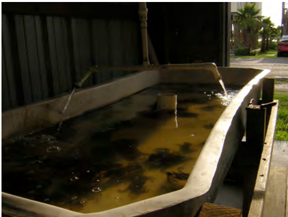
Fully utilized tank in Lyncker shed system
