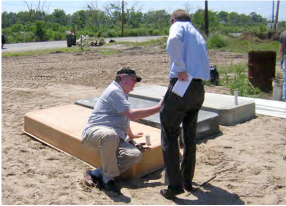
Bill Hogarth, NOAA, gluing pipe into tanks during the Gerica installation
